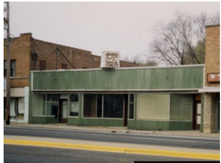
North Suburban Library District's first location on 5426 N. Second Street.
